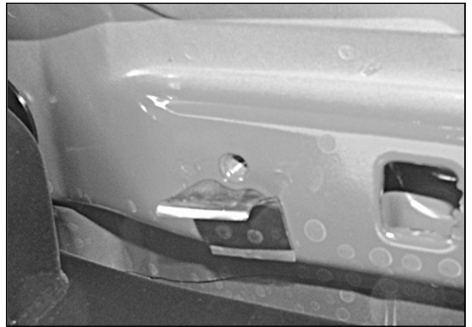
(Fig 2) M8 threaded hole in floor frame channel (passenger side-front pictured for example)
